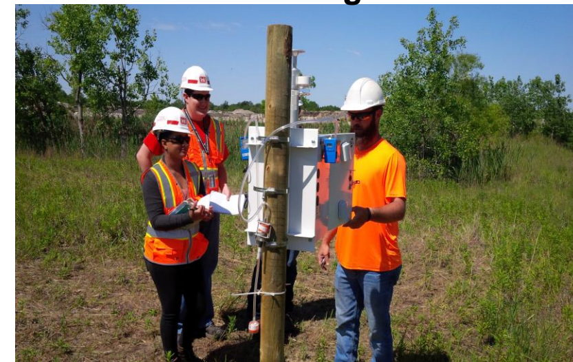
Air Monitoring Station
