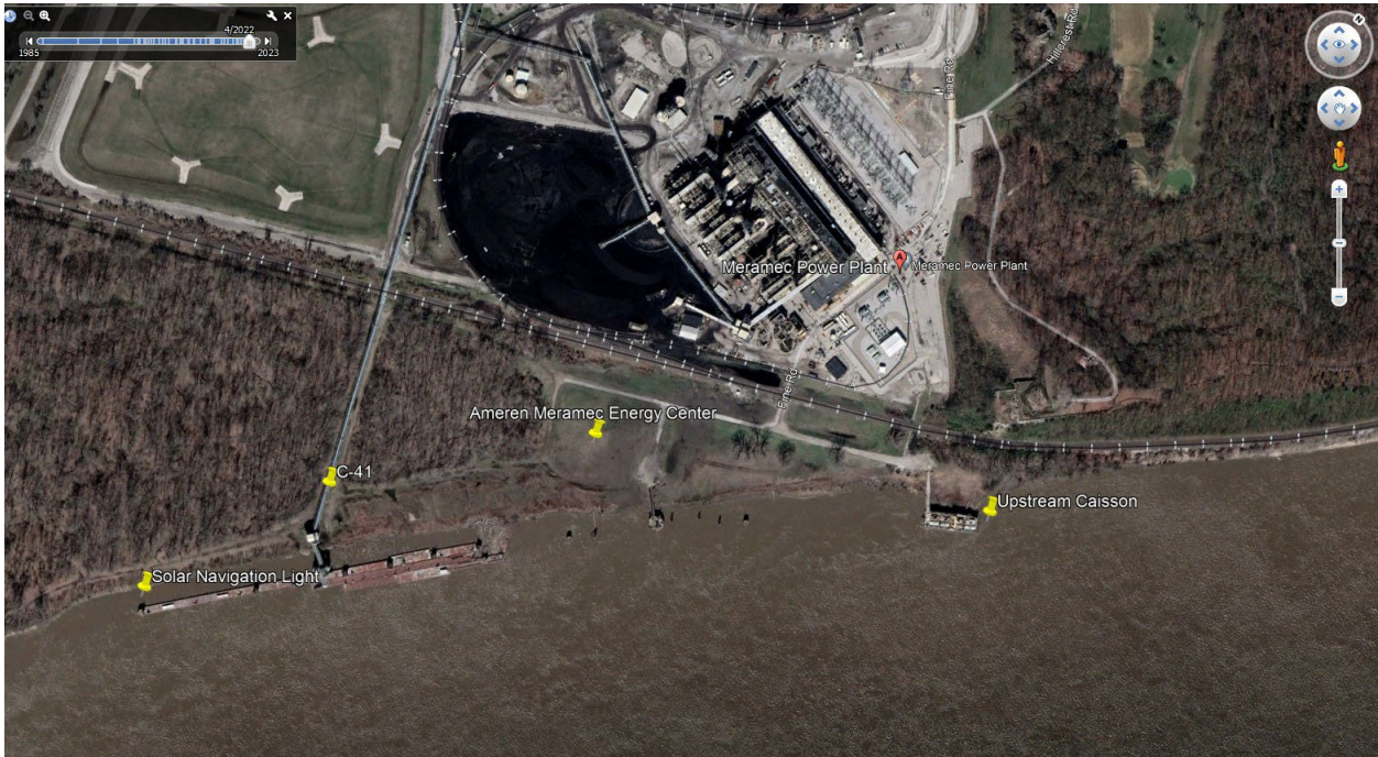
Ameren Meramec Plant (Aerial)
