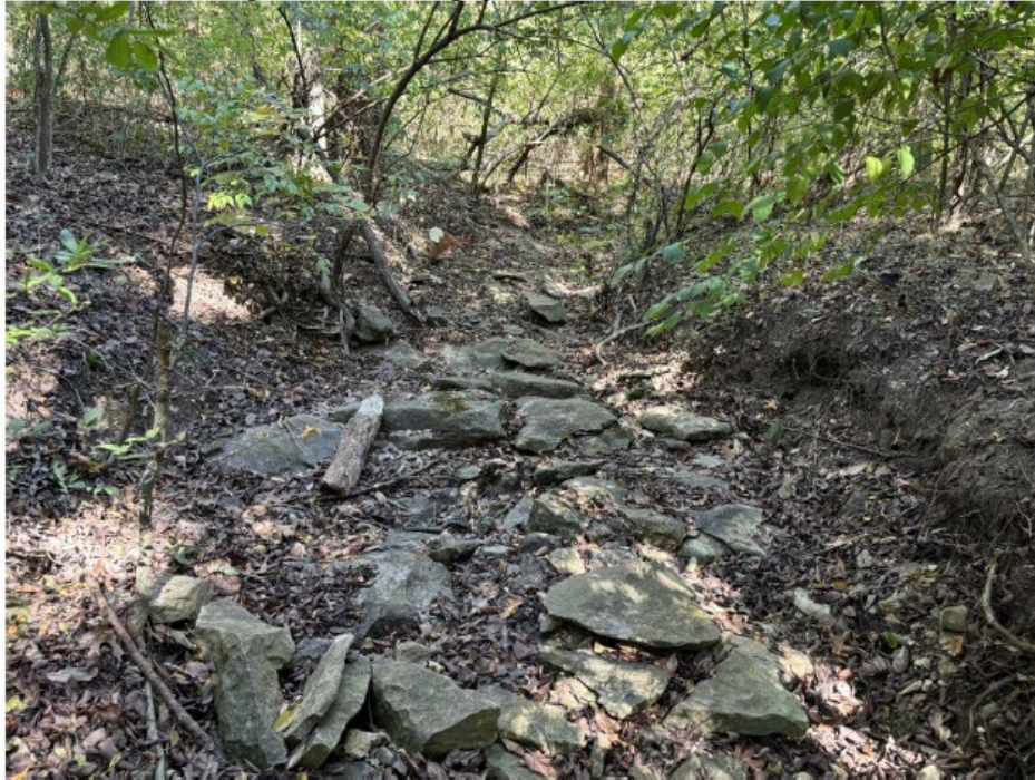
1. Overview of Drainage Feature A. facing upstream.
