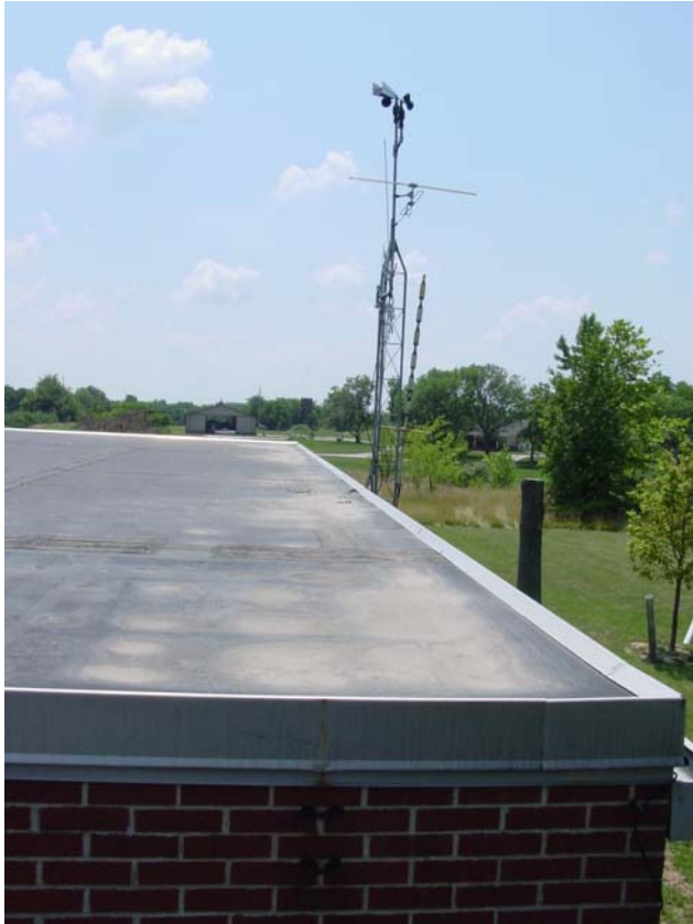
Evidence of pooling water exists in several places on the Administration Building roof
