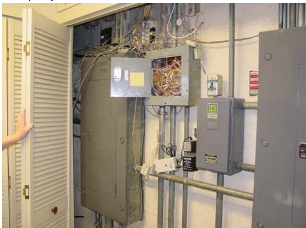
Existing wiring for electronic equipment and telephones does not have the capacity to provide the proper services needed
