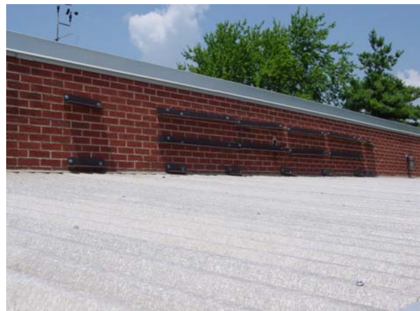
Temporary Fix for Cracked Wall
