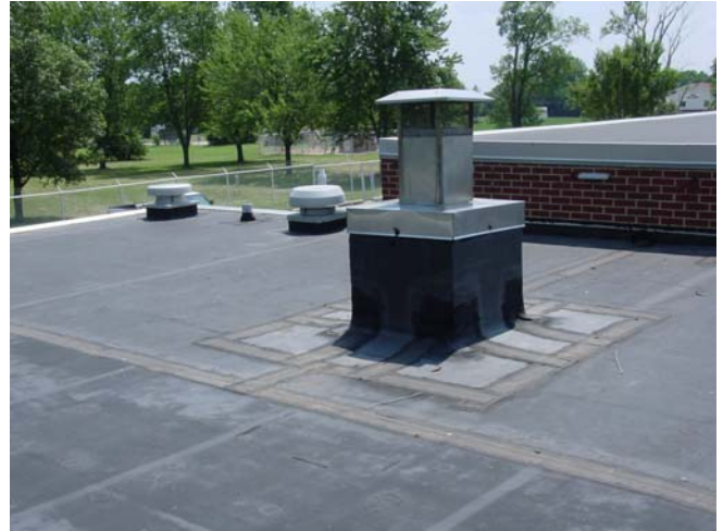
The roof has been patched in several places to stop it from leaking
