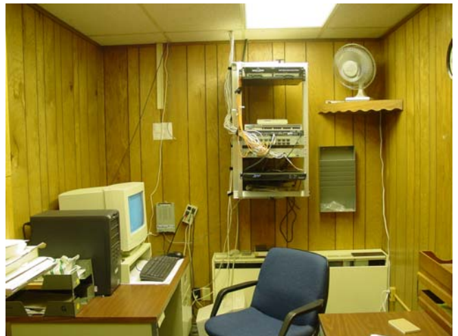
Existing wiring for electronic equipment and telephones does not have the capacity to provide the proper services needed
