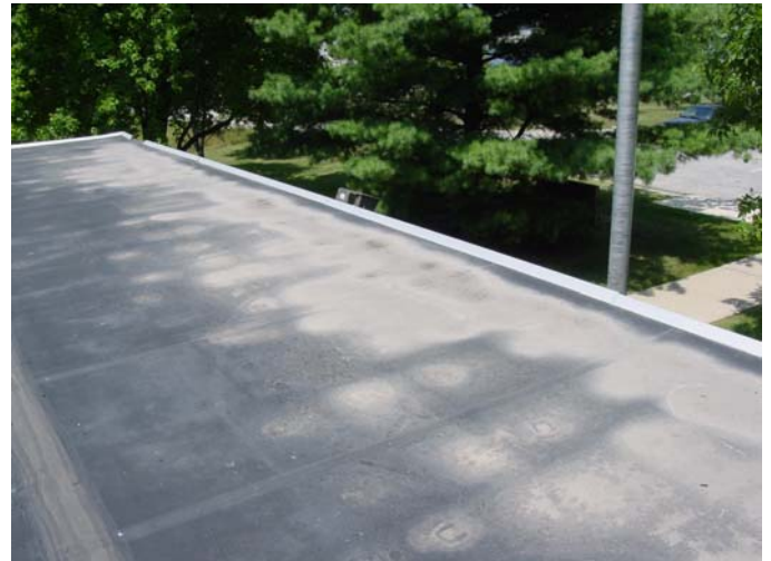
Evidence of pooling water exists in several places on the Administration Building roof
