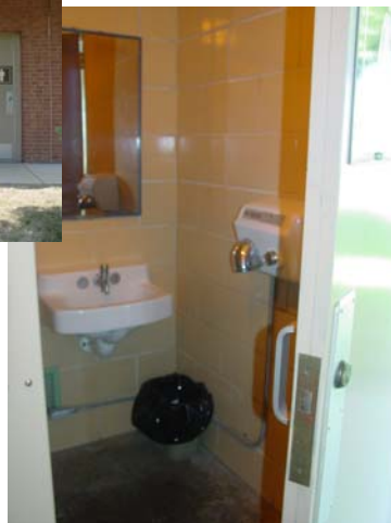
Restrooms are located outside and do not meet Uniform Federal Accessibility Standards.
