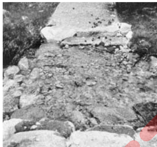
Figure 28--Wide cross drain and causeway
