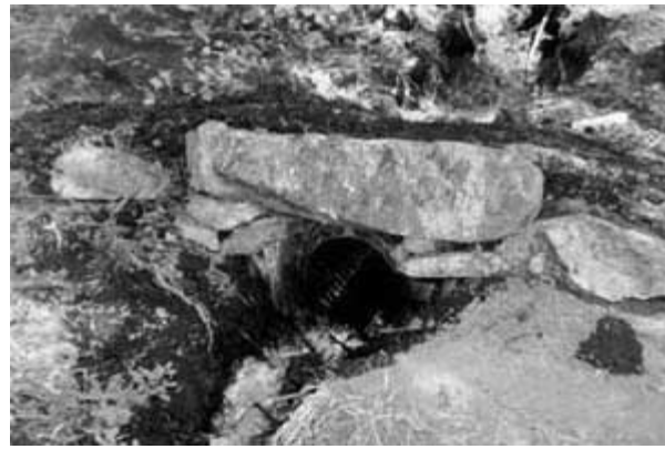
Figure 30--Culverts need to be installed at a sharp enough angle to prevent sediment from being deposited.
