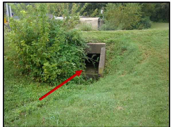
Figure 3 View of Storm Water Drain Outlet and Box Culvert Entrance near 1800 North Main Street
