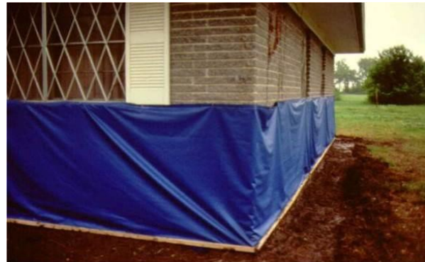
Figure 3 Temporary Dry Flood Proofing
