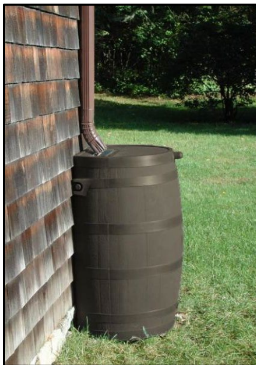
Figure 11 Rain Barrel Detention Storage
