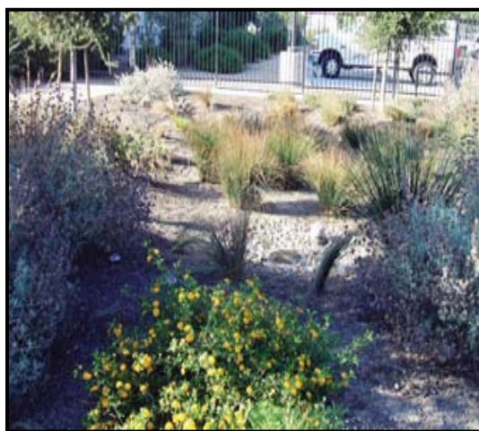
Figure 12 Rain Garden Detention Storage
