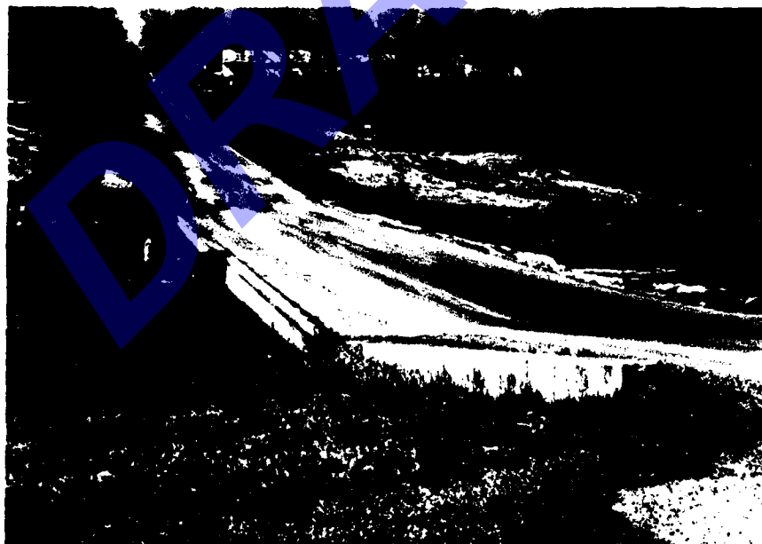
Photo 6 - View of the principal spillway drop inlet and emergency spillway broad-crested weir looking toward the left abutment.
