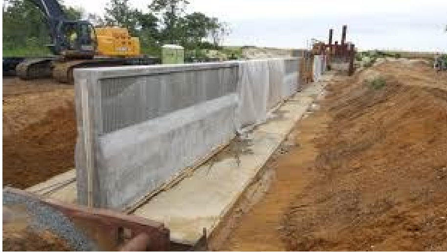
Figure 17. Floodwall (image: USACE).
