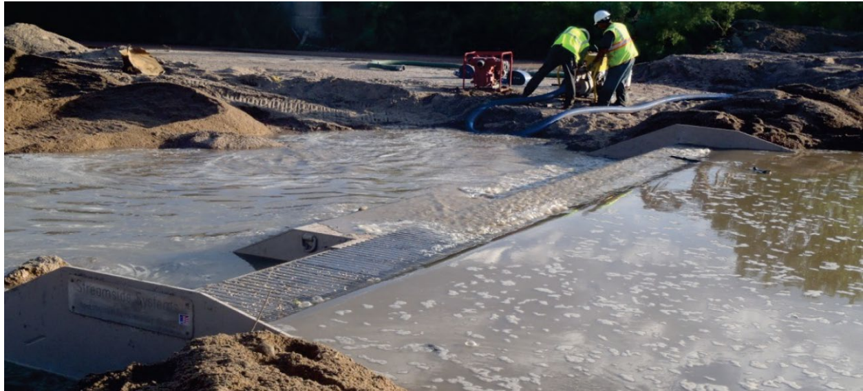
Figure 2-26: Sediment Collector During Installation, Fountain Creek, CO (Thomas, 2017)
