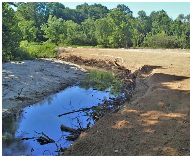
Figure 2-7: Toe Wood Immediately after Construction, LaBarque Creek, Coastal Hydrology, Inc.
