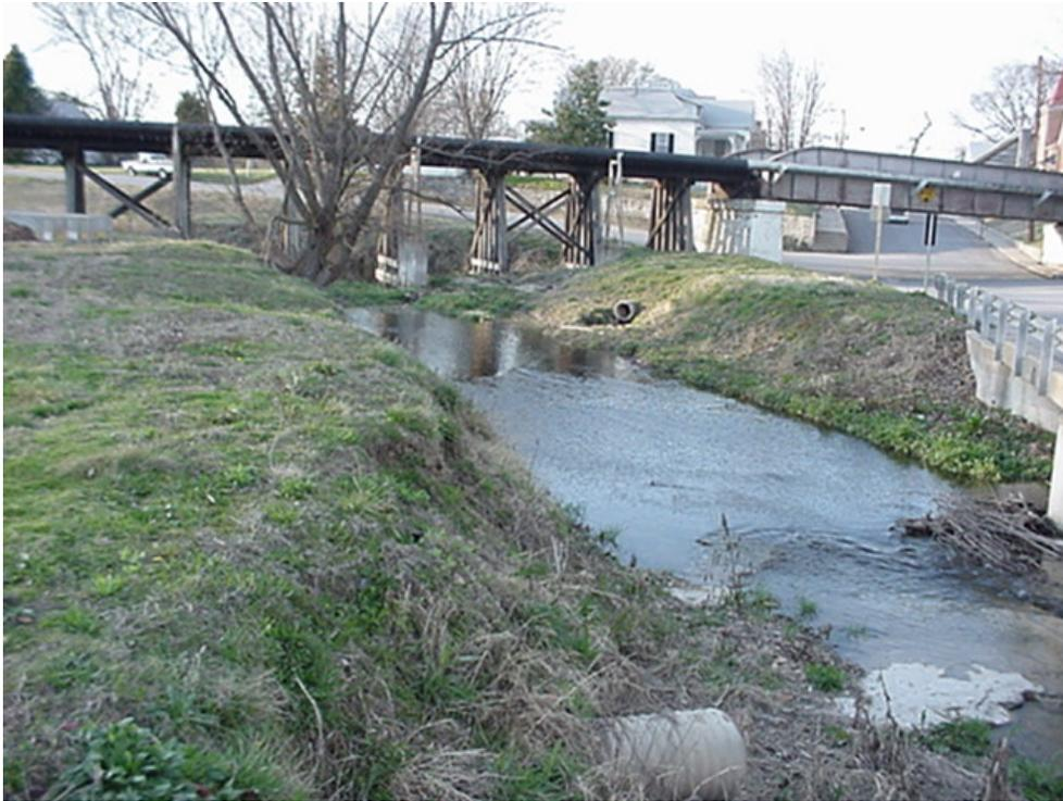
**Photo 4. South Gabouri Existing Conditions - Bridges. This old wooden railroad trestle snags debris coming down the creek, possibly contributing to flooding upstream.**
