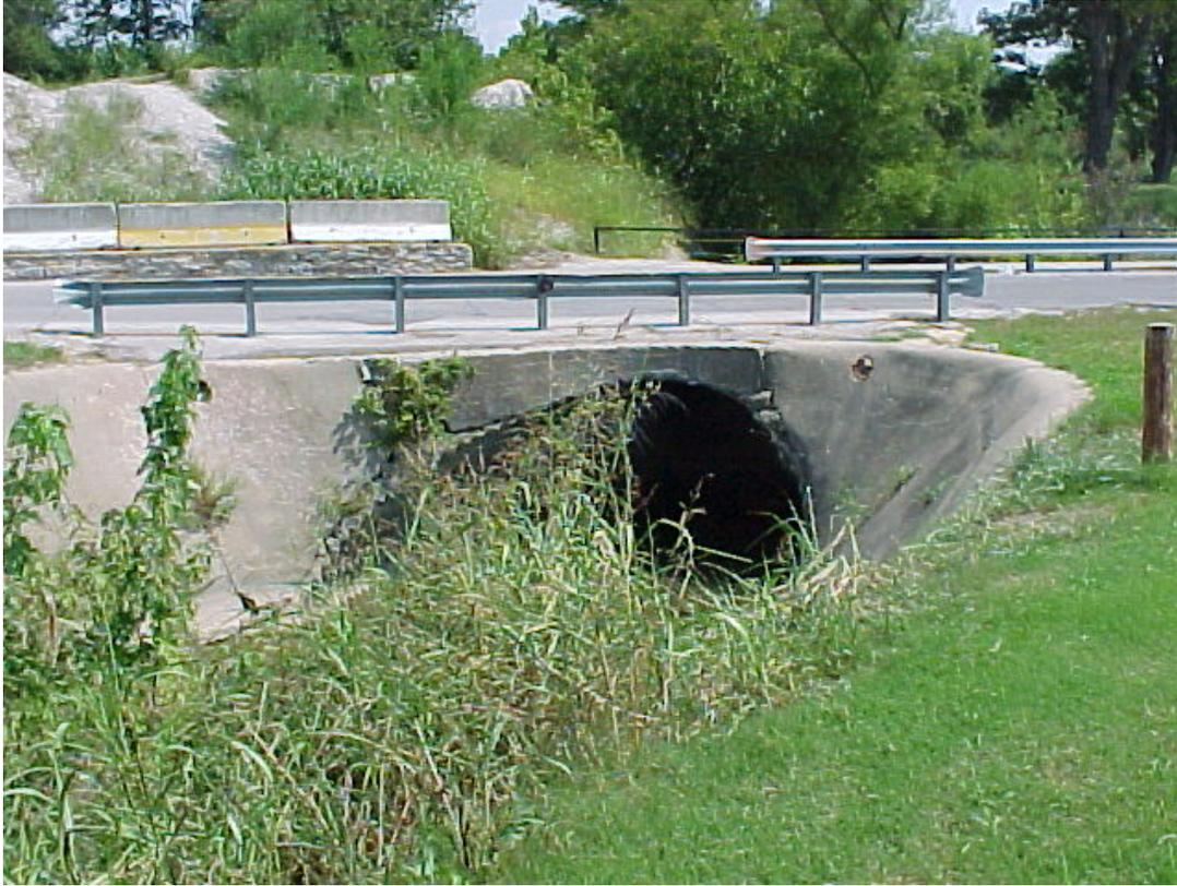
**Photo 1. North Gabouri. Undersized bridges, such as this one at Third Street, may contribute to the flooding problem.**
