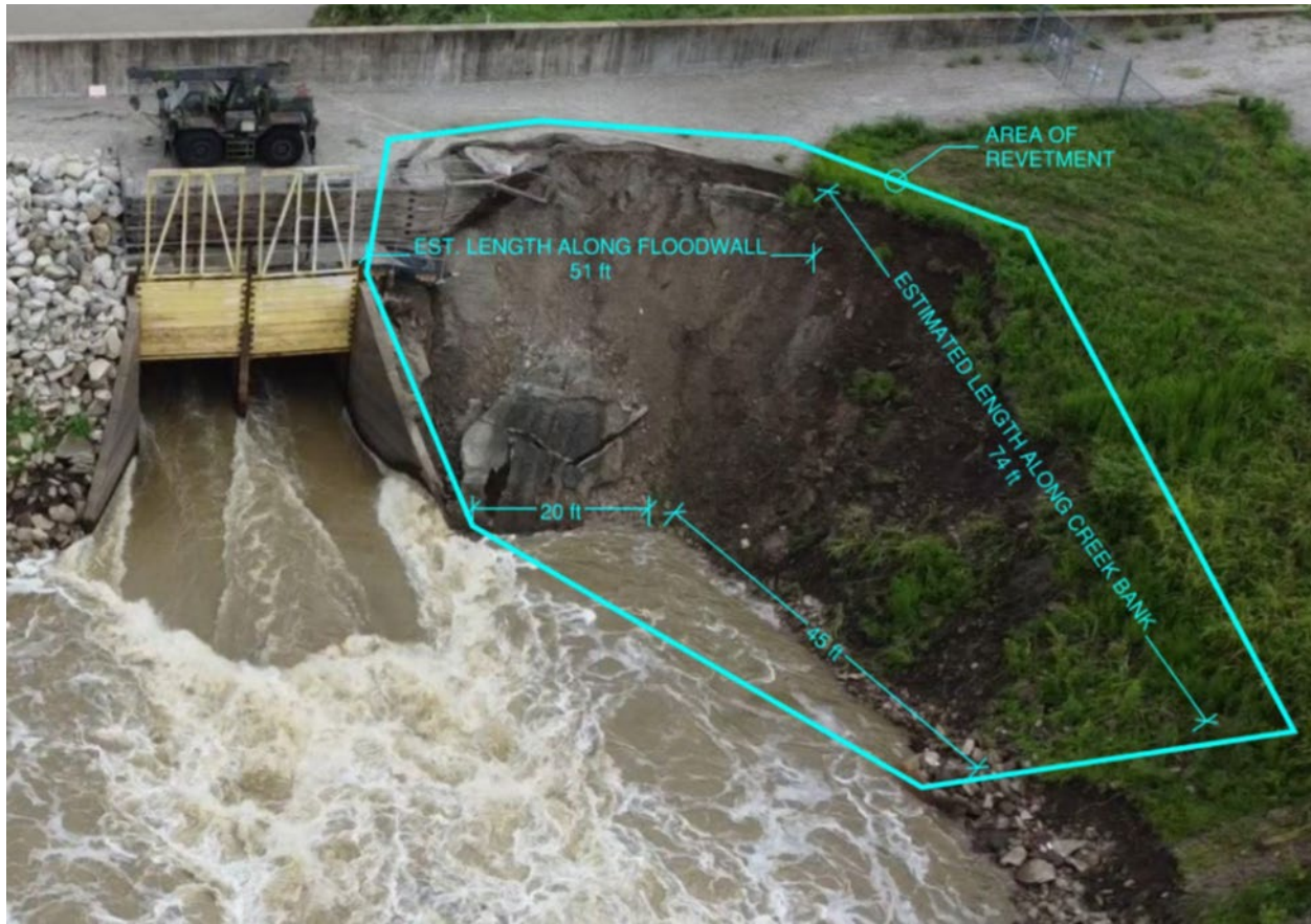
Figure 2. Scour hole in levee caused by July 2022 high water event.
