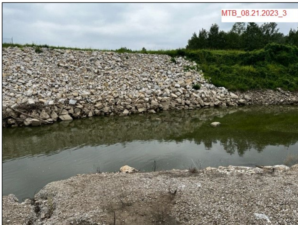
Figure 4. Levee District's repair of the eroded bank near water control structure with revetment.
