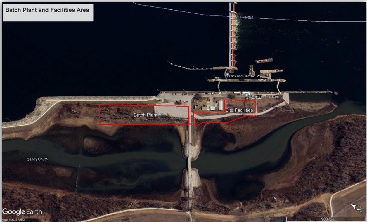
Figure 11. Batch plant and facilities area.
