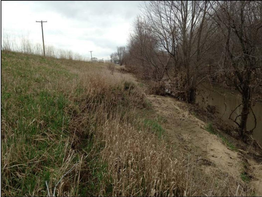
**Figure 4.** Erosion along Indian Creek at Mud Creek Drainage and Levee District.
