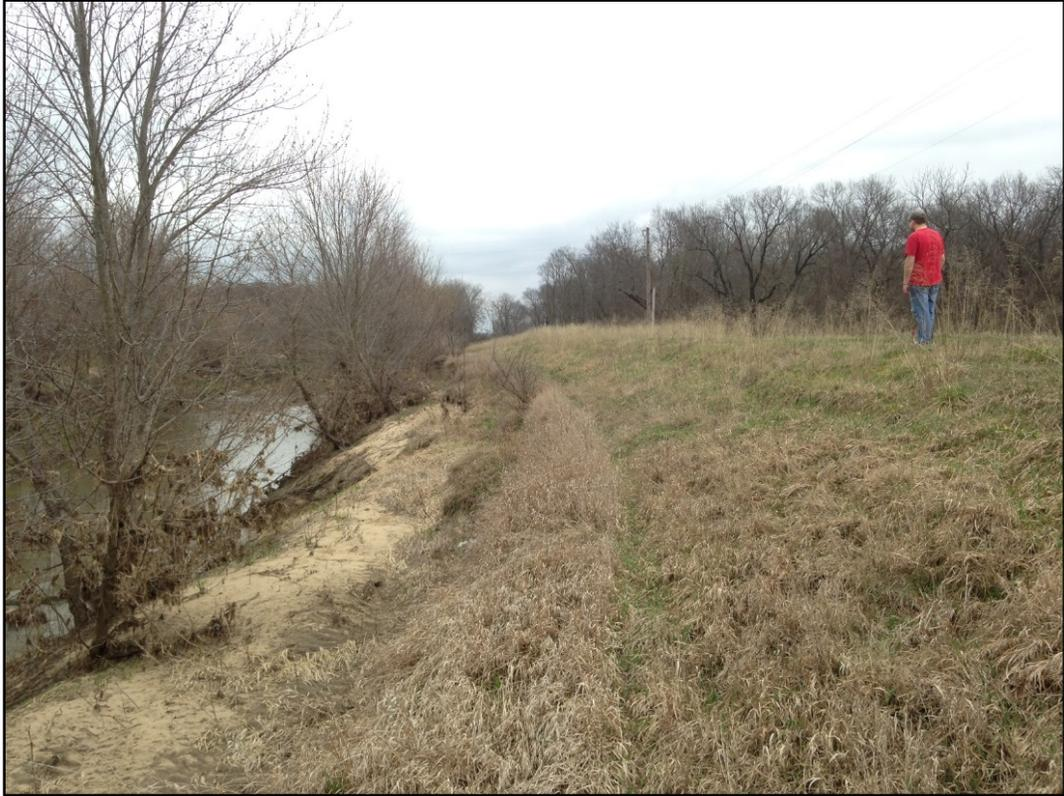
**Figure 5.** Erosion along Indian Creek at Mud Creek Drainage and Levee District.
