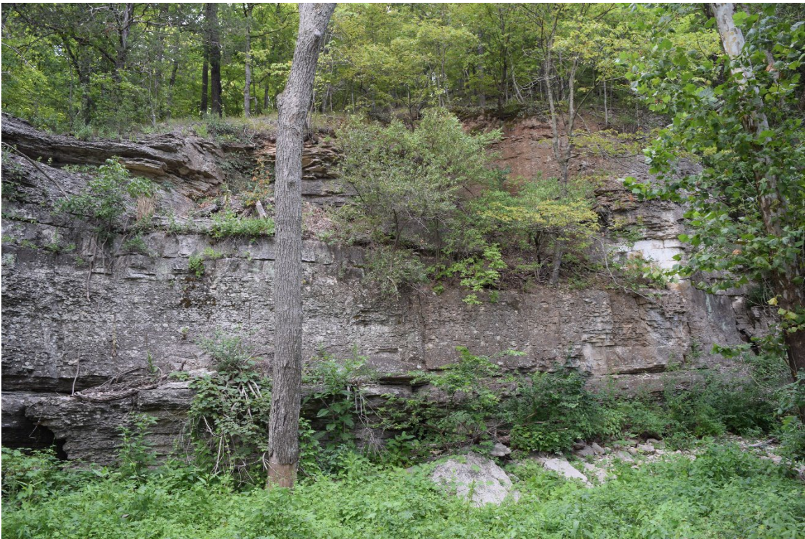
Bluff wall along eastern side of access road.
