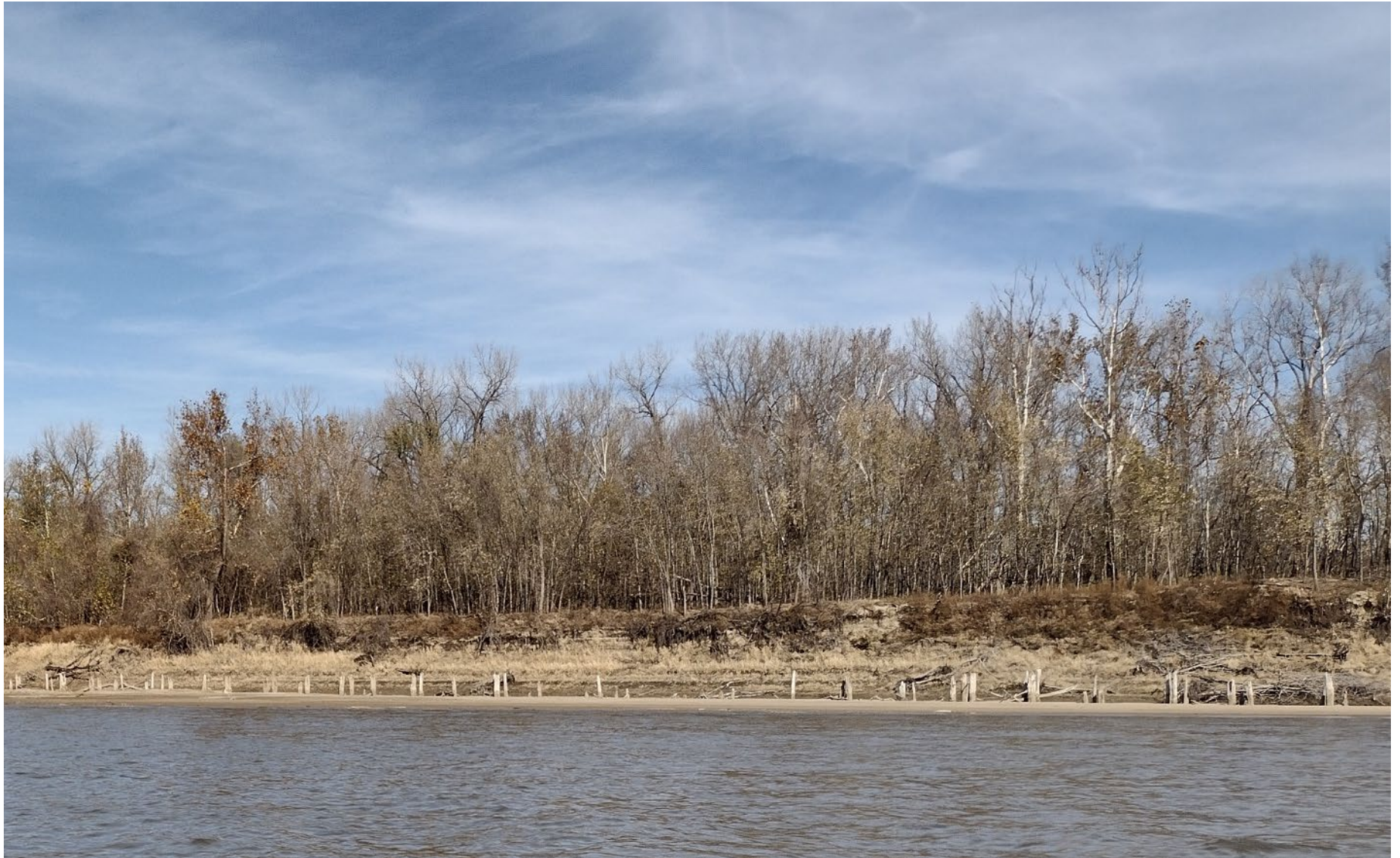
Figure 3. An existing pile dike with. Deposition has occurred within the pile dike. Photo was taken on 07 November 2022.
