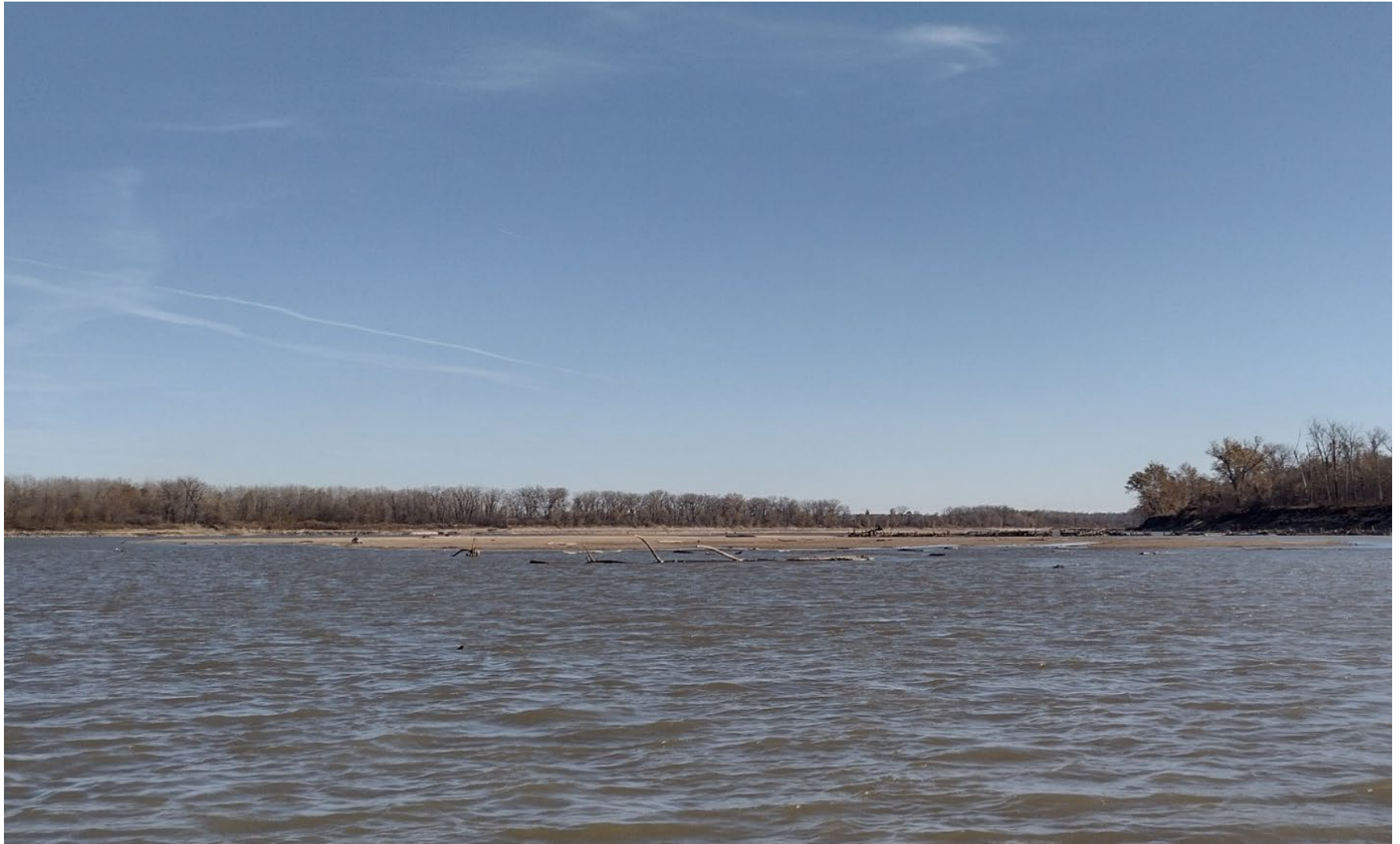
Figure 2. An existing pile dike with two or more piles constructed on the lower Missouri River. Piles are extending out of the sand by approximately three feet. Deposition has occurred within the pile dike. Photo was taken on 07 November 2022.
