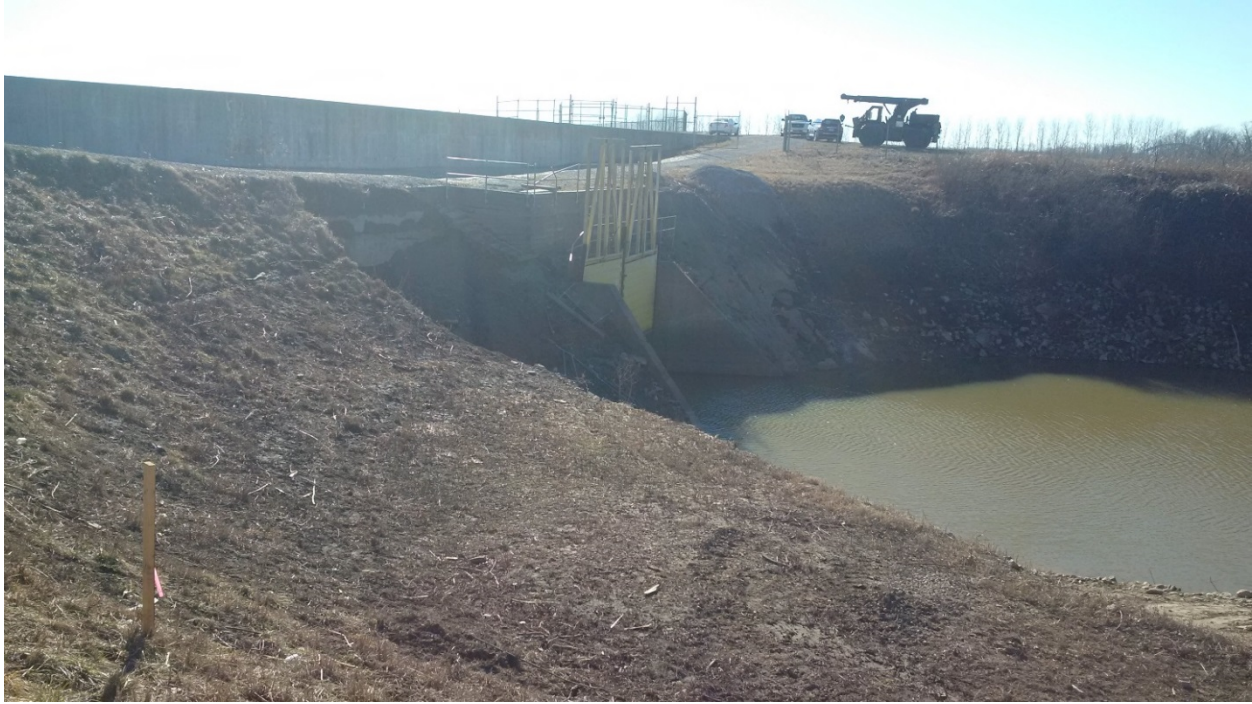
Figure 5: Standing at East End of Levee Looking West at Slope Failure Area in Levee Section, Outlet Structure with Wingwalls and Sluice Gates, and Concrete Floodwall in Background.
