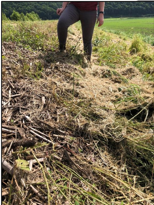
Figure 6. Example of Erosion Type I at the Bluffdale Farms Levee System.
