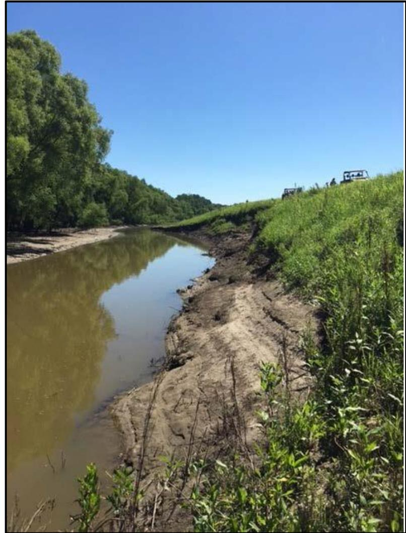
**Figure 7.** Photo of the levee slide at STA 728+20 to STA 732+40.
