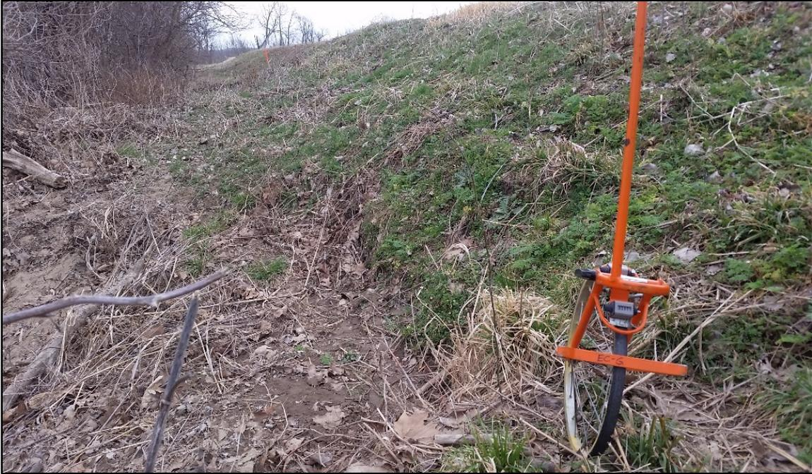
**Figure 4.** Area of erosion cause by scour approximately 300 feet long and within 7 feet of Foley levee crown.
