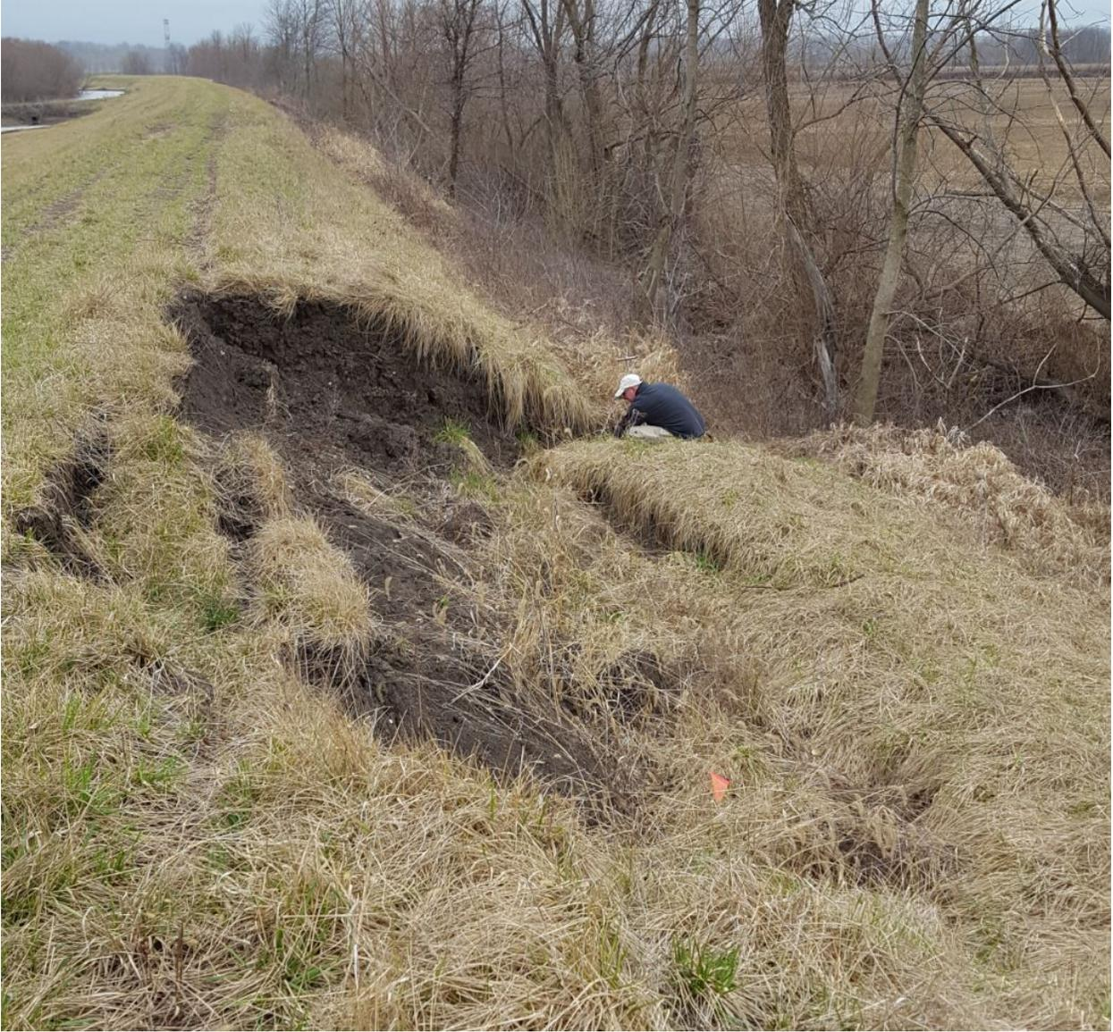
**Figure 3.** Levee slide along Cole Creek adjacent to Borrow Area 1.
