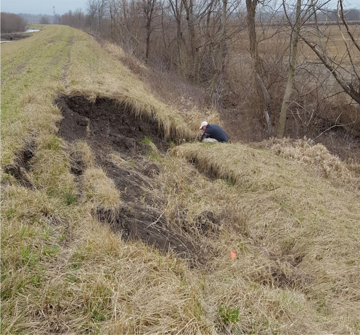
**Figure 3.** Levee slide along Cole Creek adjacent to Borrow Area 1.
