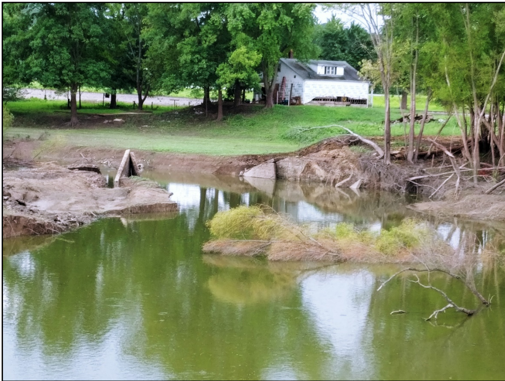
Figure 13. Ramp from the levee, damaged at Breach 1 during the 2019 spring flood.
