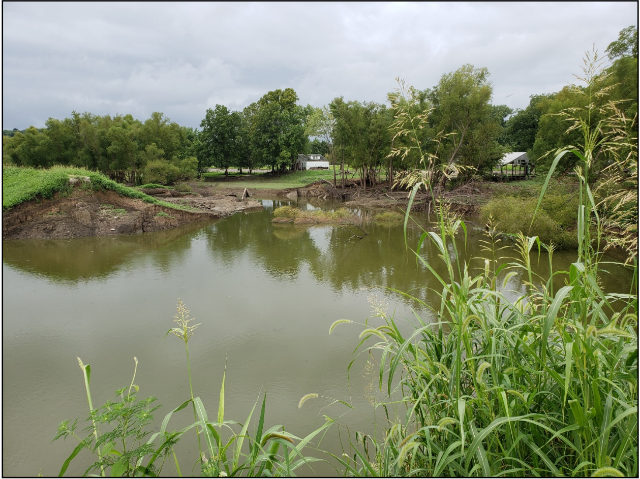
Figure 12. Photo of Breach 1 (Damage Area 10) with scour hole extending through the nearby creek. The damages occurred as a result of the 2019 spring flood at Sainte Genevieve Levee System No. 2.
