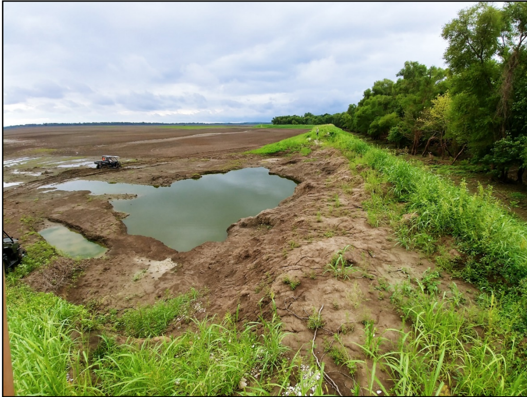
Figure 16. Photo of Breach 2 (Damage Area 11). The damages occurred as a result of the 2019 spring flood at Sainte Genevieve Levee System No. 2.
