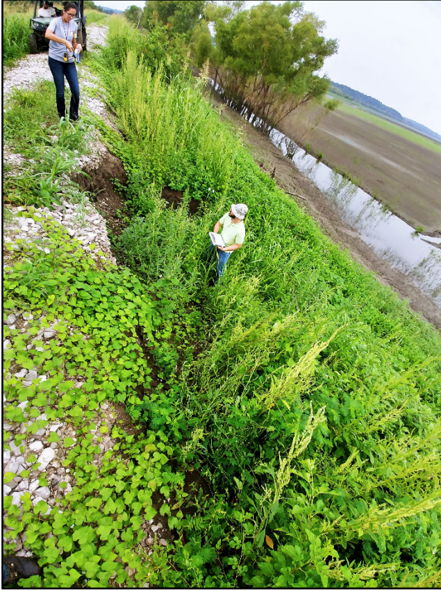
Figure 10. Example of Erosion Type III at the Sainte Genevieve Levee System No. 2.
