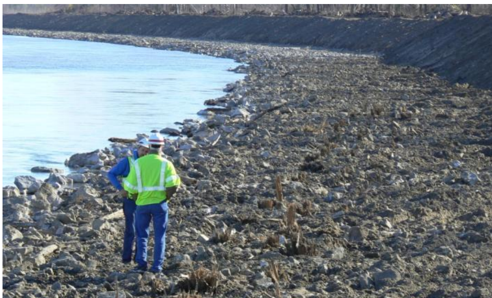
Figure H: Revetment lowering at low water, Lower Decatur Bend.
