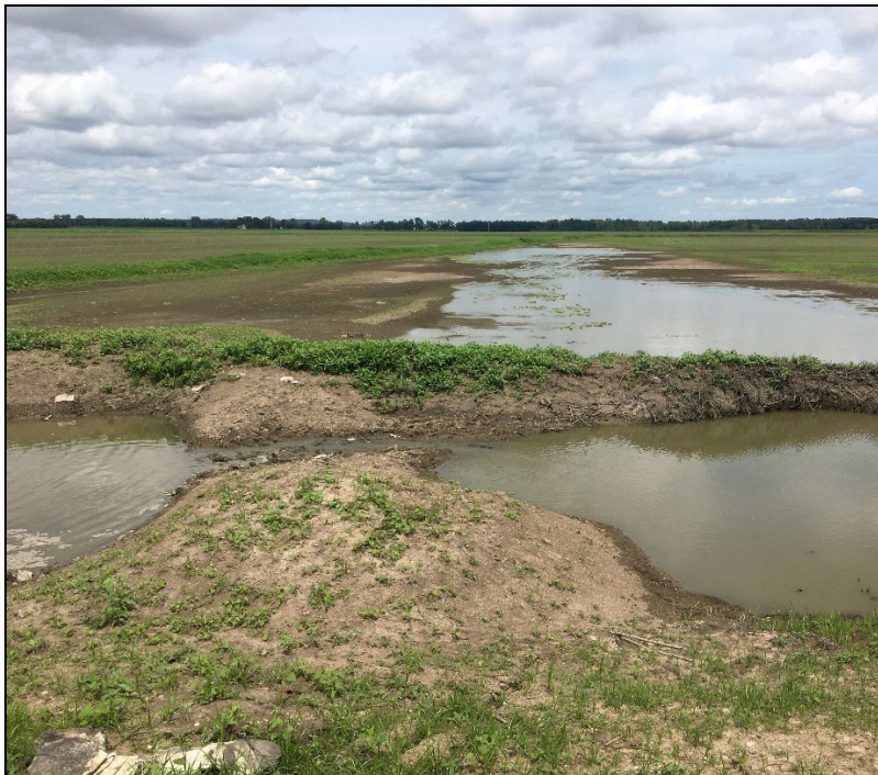
Figure 4. Photo of the breach on the Brevator Levee System as a result of the flooding event of spring 2019.
