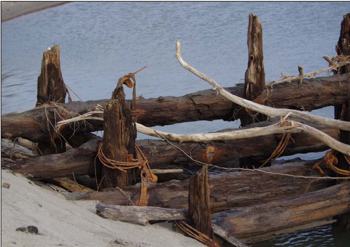
Figure 1: Remnants of timber Dike, Ste. Genevieve 2 Levee.
