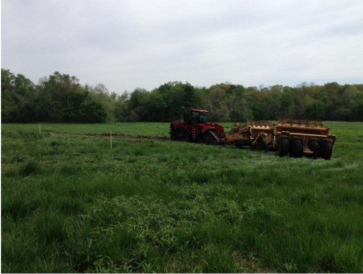
Photo 4. Example of a scraper moving material.
