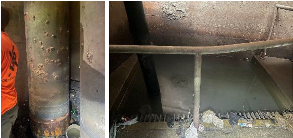
Figure 20: Corroded pump tube and sump clogged with trash/debris at Parkside pump station. July 2022 (Photo courtesy of USACE)
