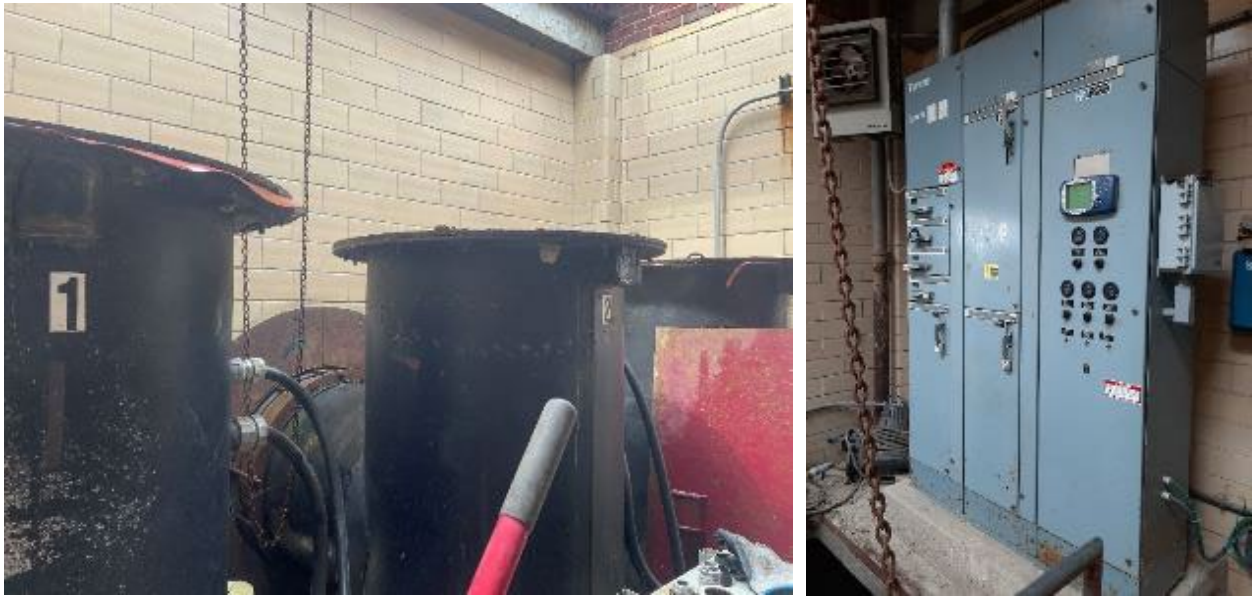
Figure 19: Pump tubes and electrical motor control center (MCC) on operating floor at Parkside pump station. July 2022 (Photo courtesy of USACE)
