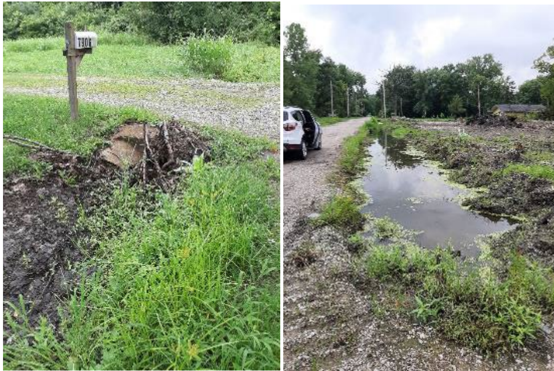
Figure 24: Damaged culvert and sedimented local drainage ditch. July 2022 (Photo courtesy of USACE)
