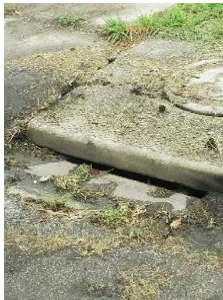
Figure 16: Blocked storm sewer inlet July 2022 (Photo courtesy of USACE)
