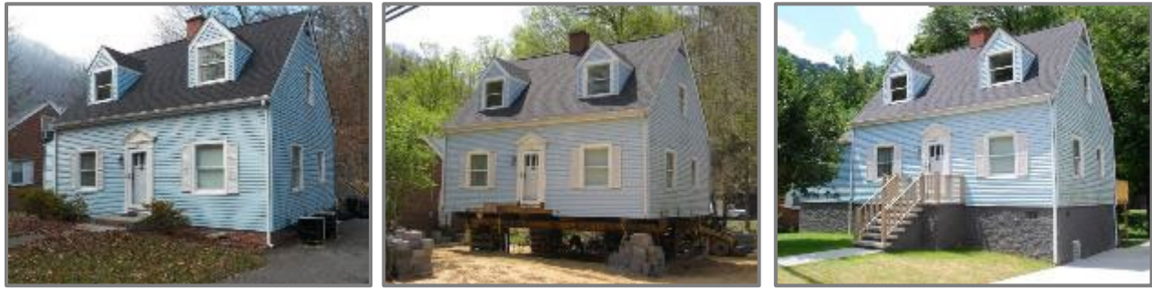
Figure 29: Elevation of a Residential Structure. Image- USACE
