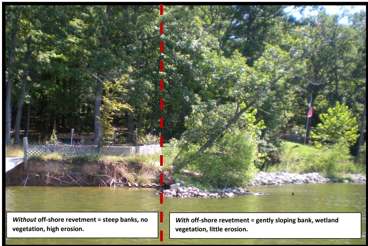
Photo 1: Portions of lake with no revetment (left side) and off-shore revetment (right side).
