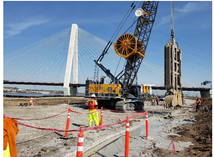
Figure 1: Construction of cutoff wall, completed in October 2022
