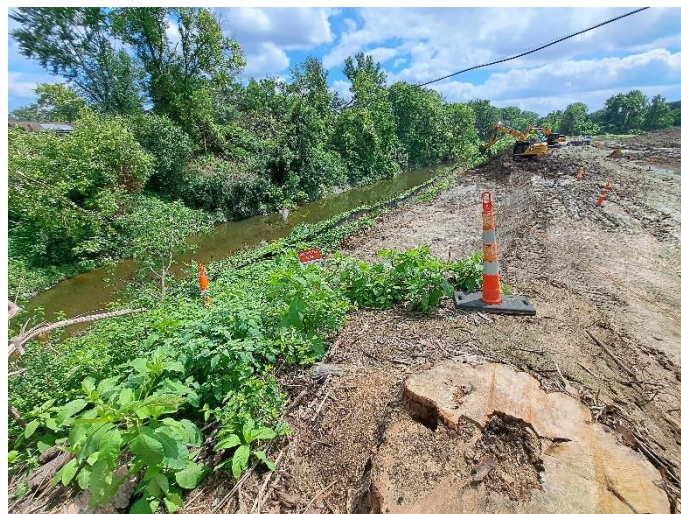
Figure 1: Remedial Activities at Coldwater Creek
