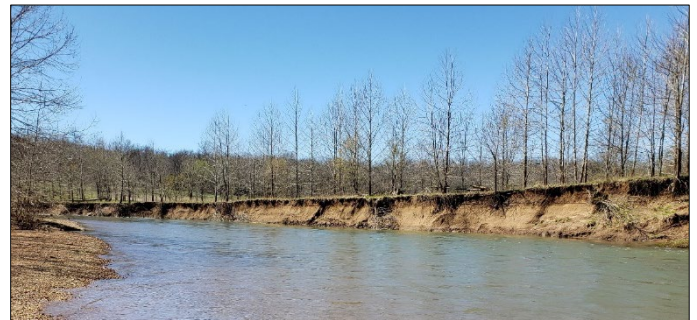
Unstable banks along the Big River continue to contribute excessive sediment and heavy metals to the aquatic ecosystem.
