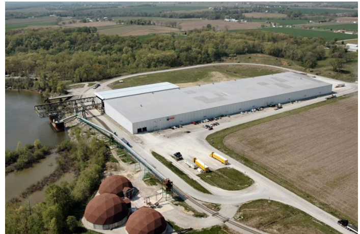
Aerial view of KRPD Terminal 2.
