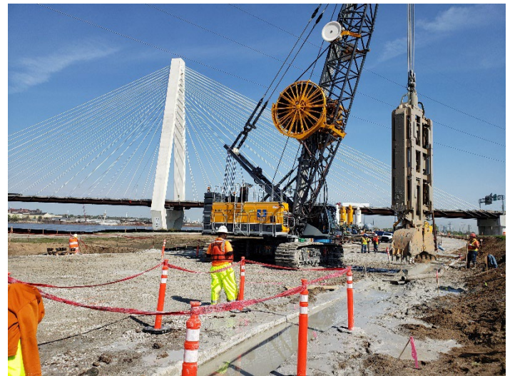
Construction of cutoff wall, completed in October 2022
