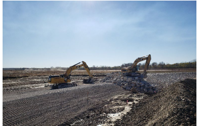
Dogtooth Bend Overflow Structure Construction (completed Jan 2021)
