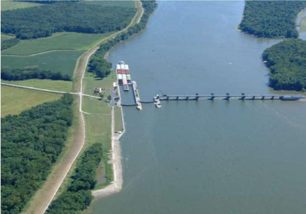
*UMR Lock and Dam with single 600ft lock chamber.*
