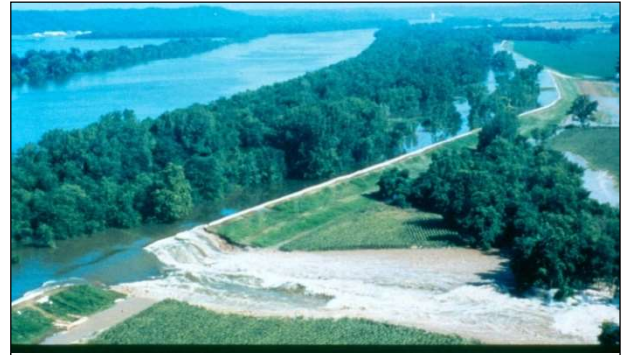
Levee overtopping with breach during 1993 flood.
