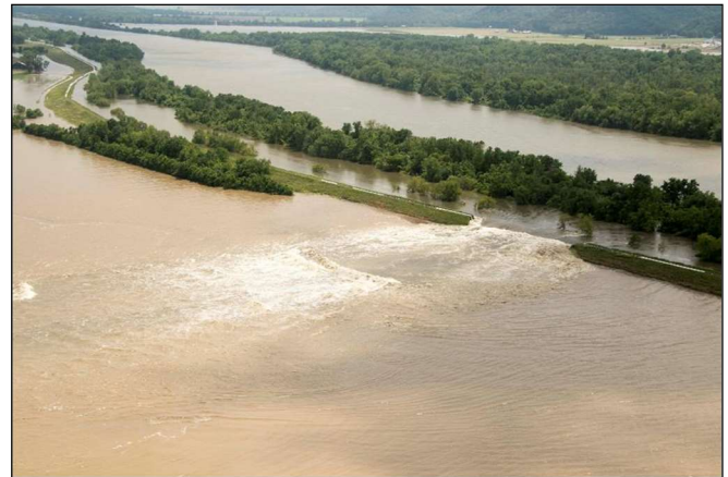
Levee overtopping with breach during 2019 flood.
