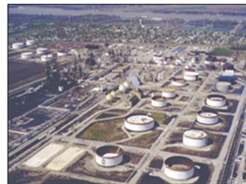
Critical infrastructure includes the Wood River Refinery
