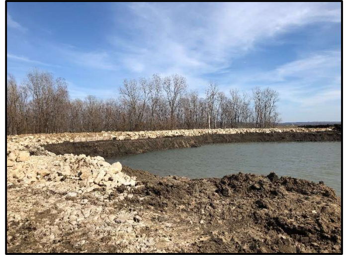
Start of breach repair at Elsberry MO, March 2020.
