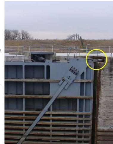
**Locks 27 damaged embedded metals, high risk regionally identified backlog maintenance, funded in IJA, FY22.**
