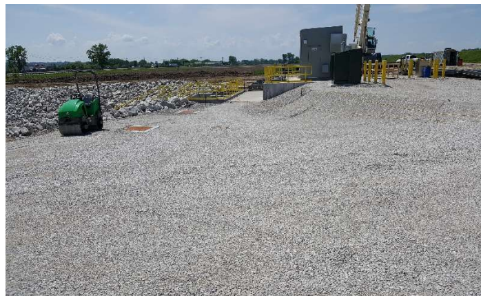
Watershed 4 pump station construction.
