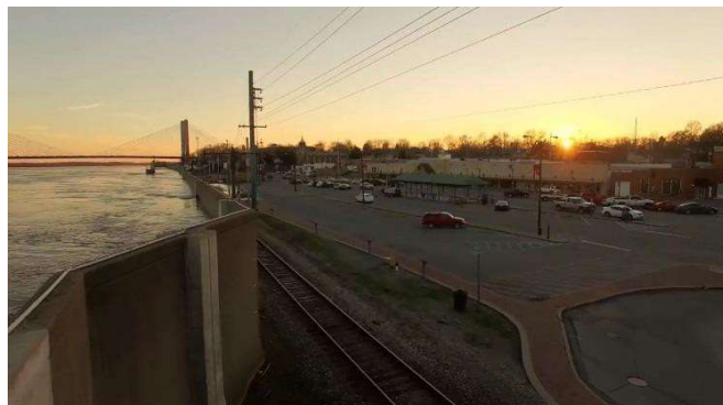
Cape Girardeau floodwall.
