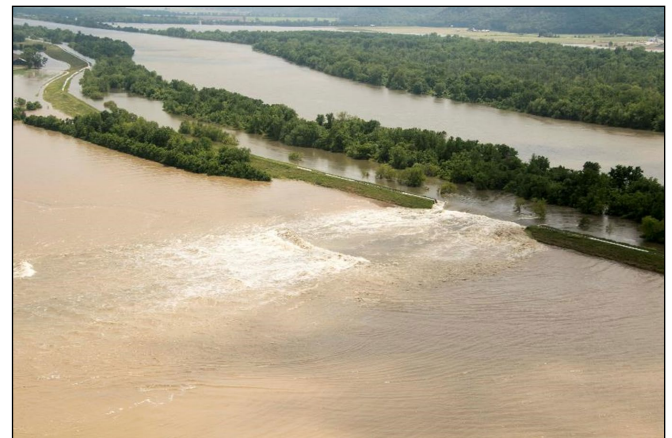
Levee overtopping with breach during 2019 flood.
