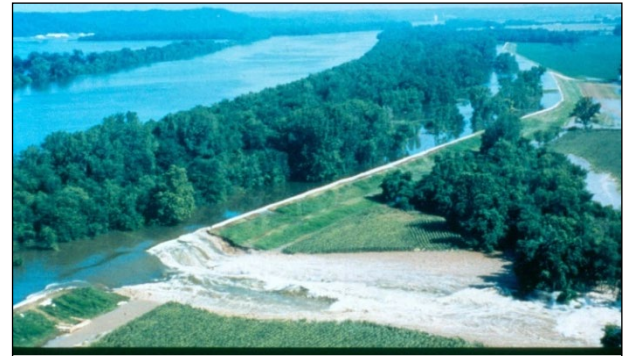
Levee overtopping during 1993 Flood
