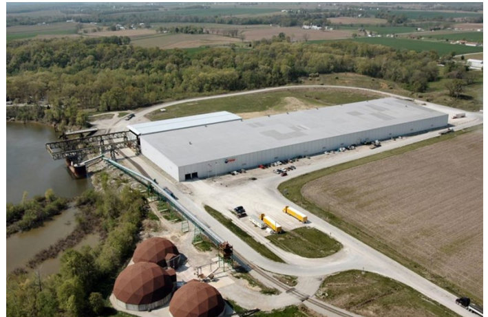
Aerial view of KRPD Terminal 2.
