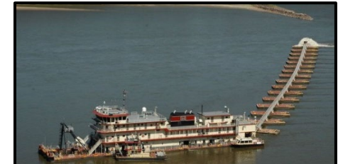
The Dredge Potter working critical routine dredging at Illinois River mi 77
