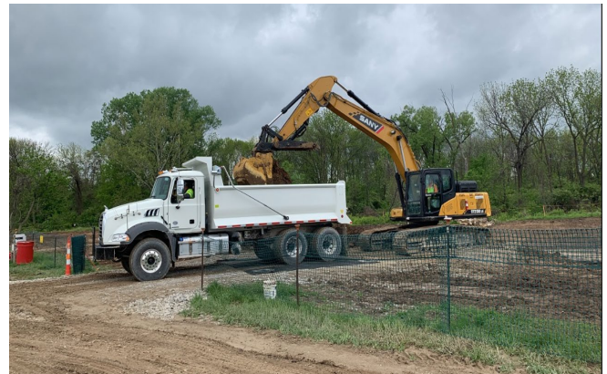
Remedial activities at the Former Ballfields area of SLAPS VPs.
