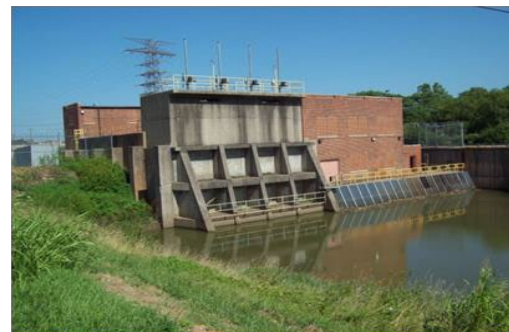
MESD north pump station.
