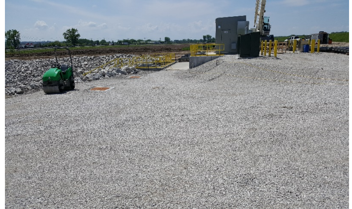
Watershed 4 Pump Station Construction.
