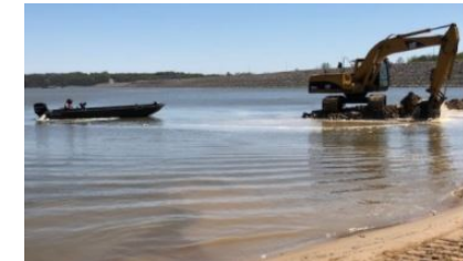
Dam West Beach Scour Repair
