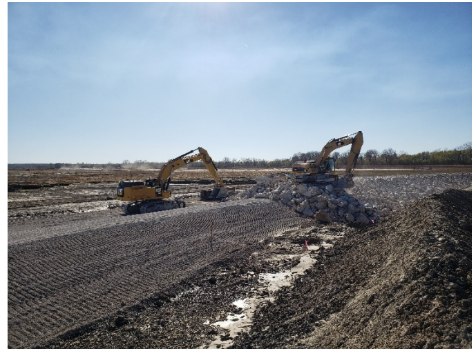
Dogtooth Bend Overflow Structure Construction (completed Jan 2021)
