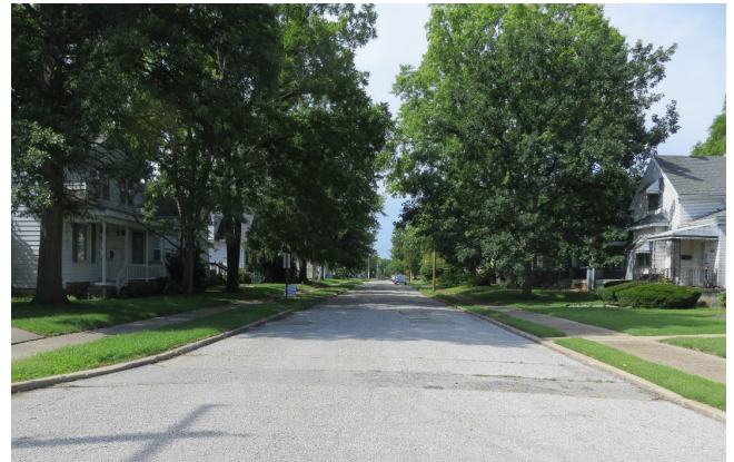
Example of Neighborhood Served by New Storm Sewer Line
